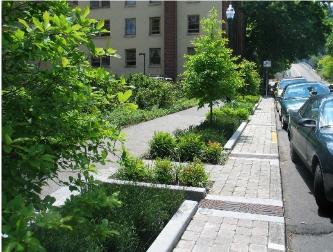
Example of Green Infrastructure Infiltration Planter
